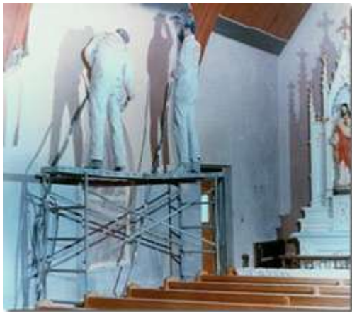
Cracked plaster walls sealed with light rose tinted Cocoon
