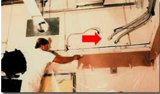
Sheet metal dust isolation plenum - note pipes
