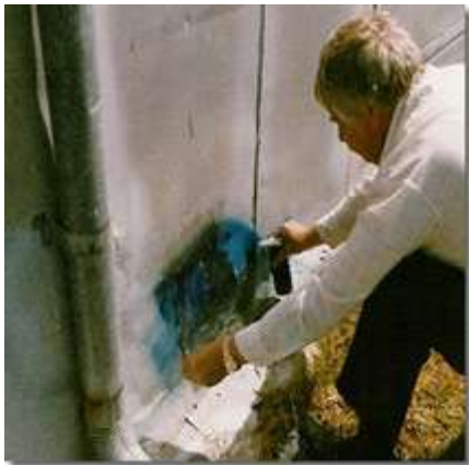
Tabacco fumigrant barn has a leak
