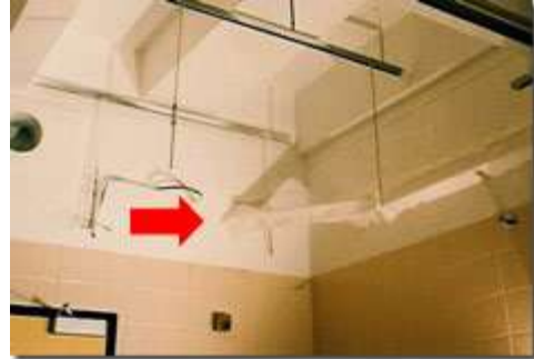
Sheet metal dust isolation plenum - note pipes
