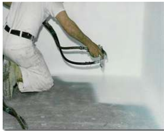
Overlapping Cocoon onto floor ensures a complete seal.
