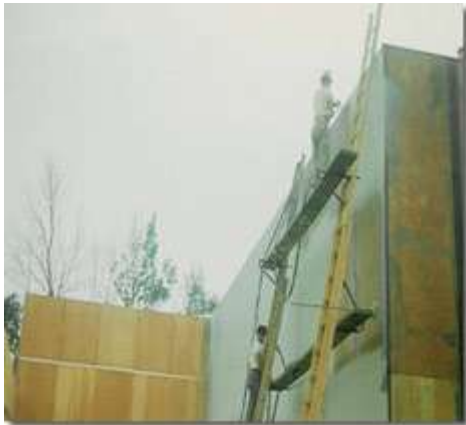
Plywood apple storage facility sealed with Cocoon.
