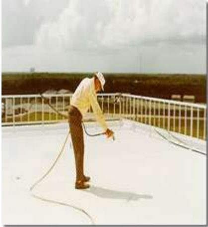
Applying Cocoon to the Vertical Assembly Building and Launch Control Center - NASA
