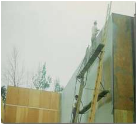
Plywood apple storage facility sealed with Cocoon.
