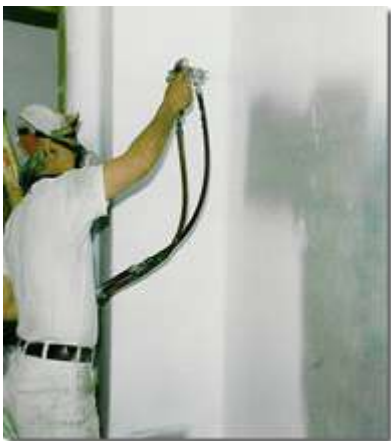
Attention to corner detail.
