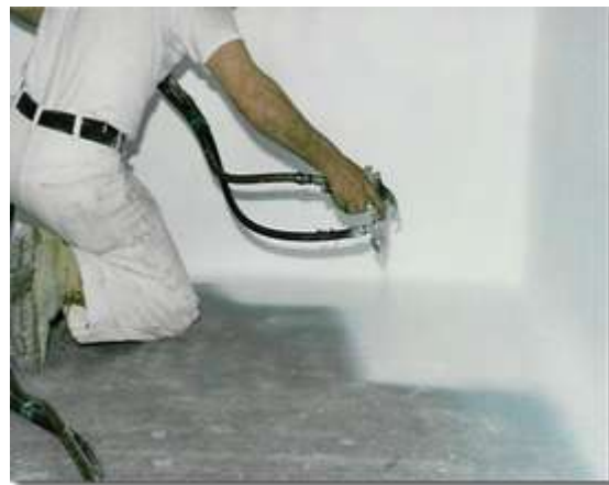
Overlapping Cocoon onto floor ensures a complete seal.
