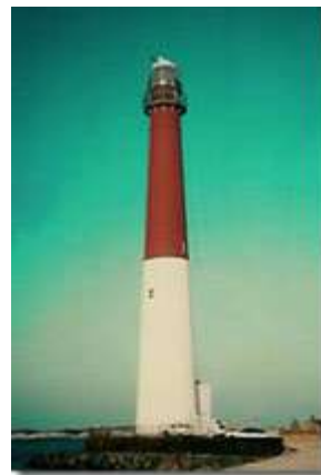
A lighthouse with a metal roof & brick walls with Cocoon.
