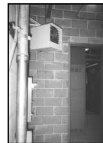
Freeze/moisture protection in a generator vault
