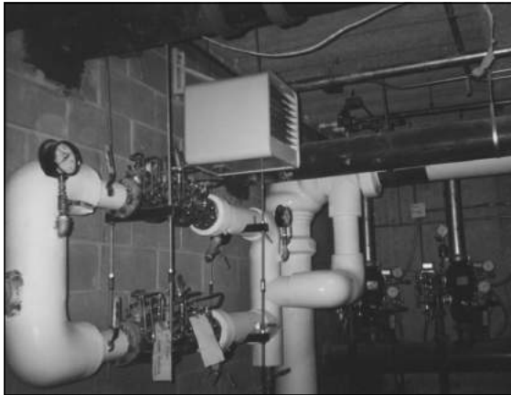
Water pumping and treatment room, protected from freezing and humidity with King KB unit heater
