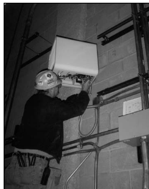
A unit heater being installed in a Chicago high rise electrical room for humidity and freeze protection
