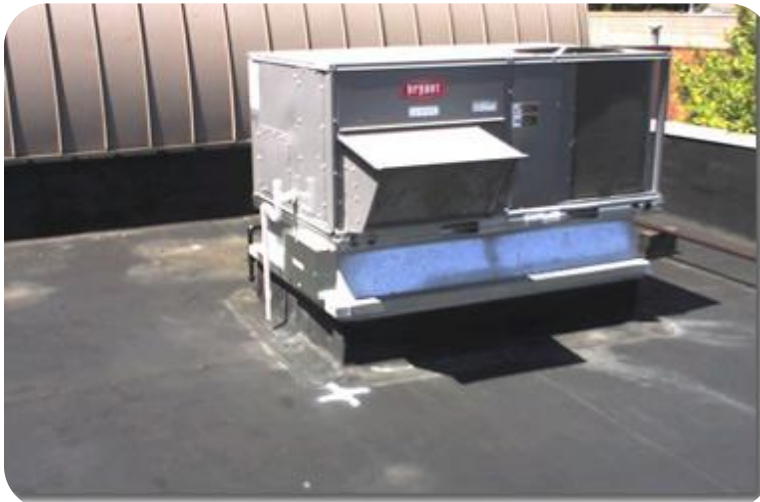
The base of the roof at this time has not been coated with Polarroof RAC.
