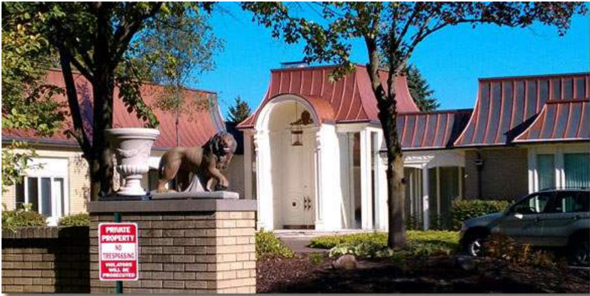
Work in progress - Home in Grand Blanc, MI
