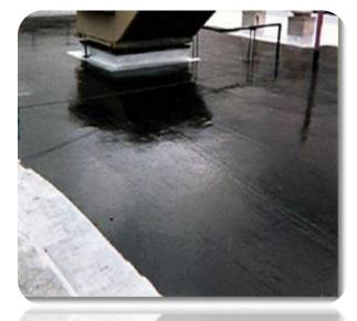
ROOFDX SUPER has been used to embed the ROOFAB here on a concrete roof deck. The top coat is POLAROOF RAC (silver).
