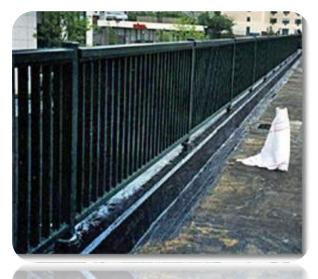
Here, ROOFDX SUPER and ROOFAB has been used to provide a waterproof membrane to the concrete curb. Andek POLAJOINT was used to set and seal the posts.
