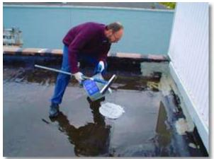
Here we had a leak on a smooth surface, modified bitumen membrane. After the excess water was swept away, RUBBERKOTE 1047 was applied and spread over the general area.
