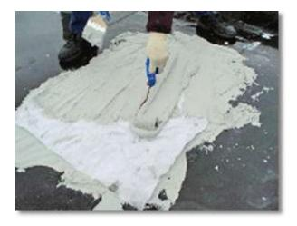
The excess RUBBERKOTE is rollered in or squeegeed  $into\ the\ ROOFAB.$
