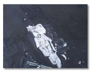
Using a brush, roller, squeegee or combination of all, lay ROOFAB as reinforcement and saturate fully.
