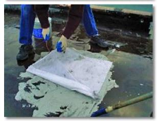
When the general area is covered, a piece of ROOFAB is cut and laid into the RUBBERKOTE 1047 as  ${\rm reinforcement.}$
