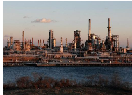
Sun Oil Refinery Philadelphia, PA USA
